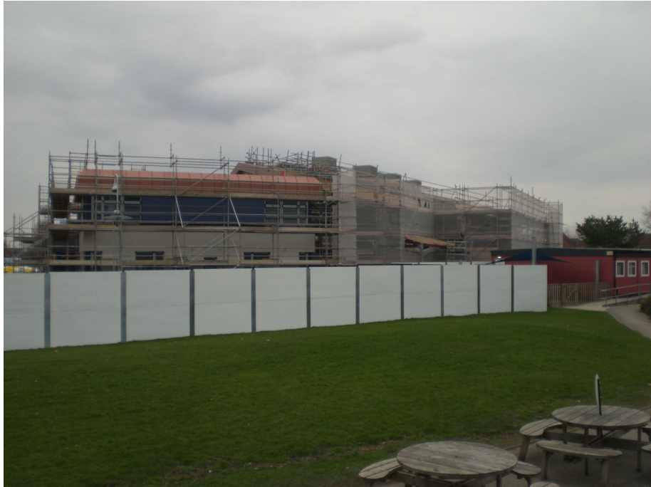
Progress being made with the new Clifton with Rawcliffe Primary School
